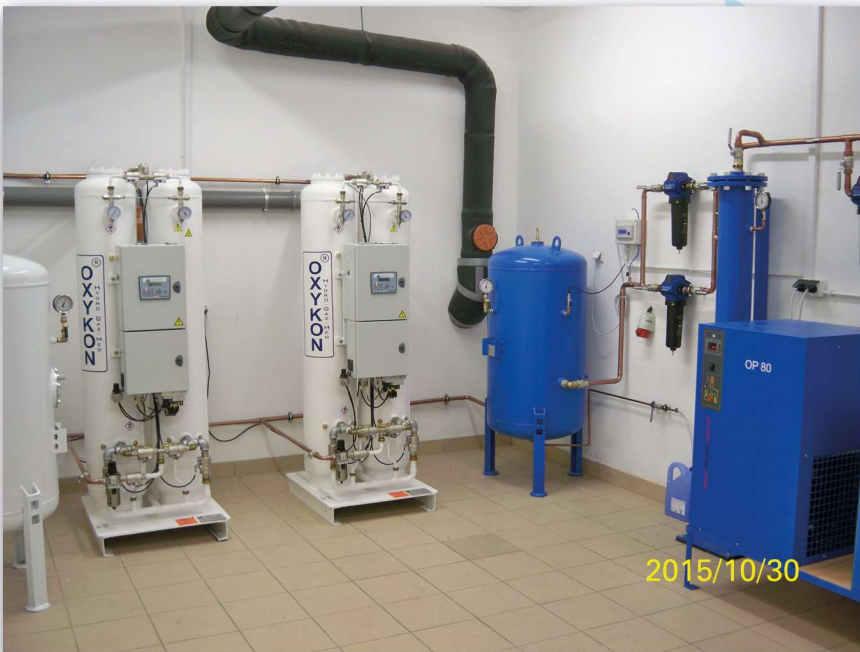
Oxygen concentrator system
