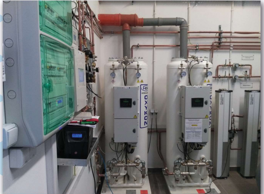
Oxygen concentrator system
