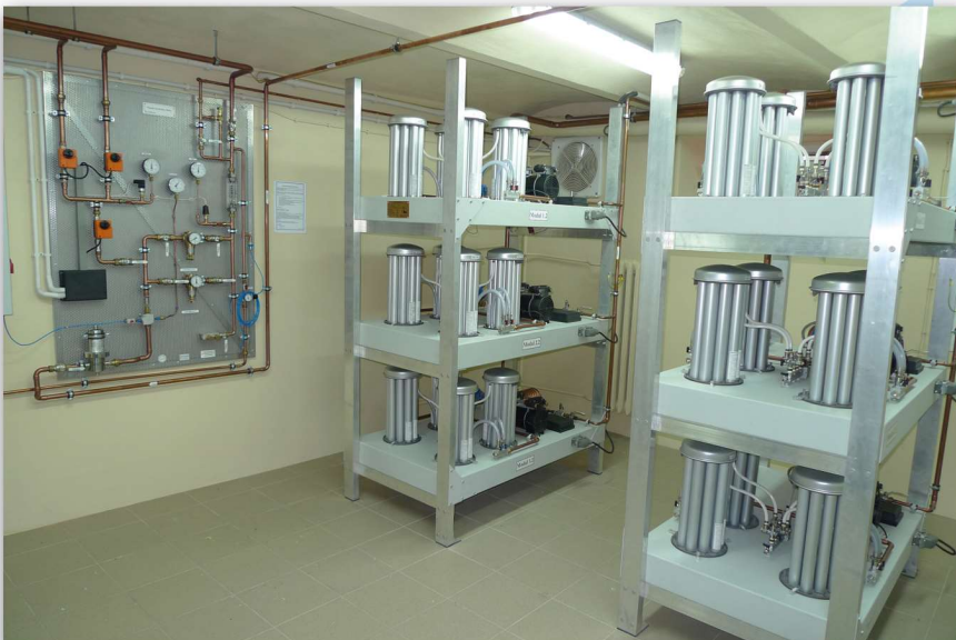
Oxygen modular concentrators system
